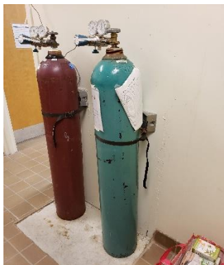
Cylinders secured to a wall.
